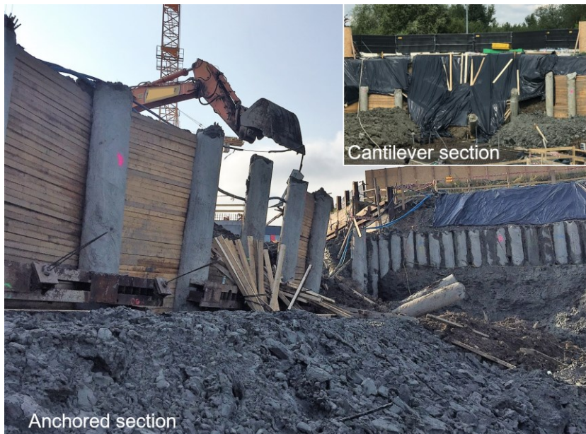
Fig. 1. View of the collapsed sections of soldier pile wall.
