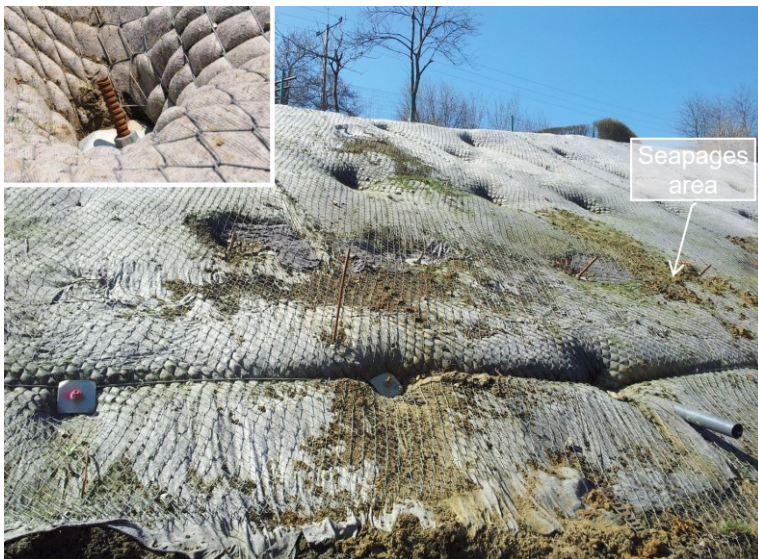
Fig. 5. General view of the deformed slope with detail of the overtensioned soil nail and steel mesh.
