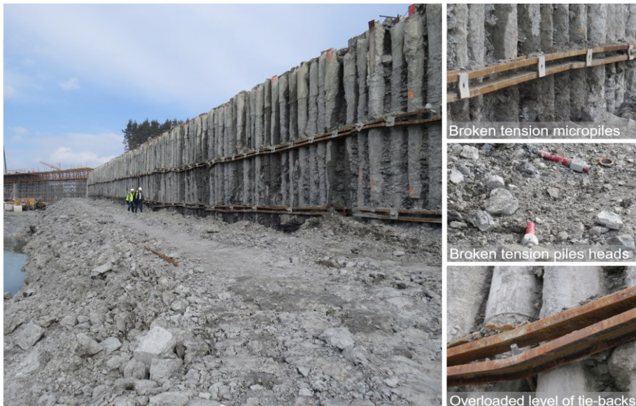
Fig. 6. General view of the construction with emergency abutment and details of damaged elements.
