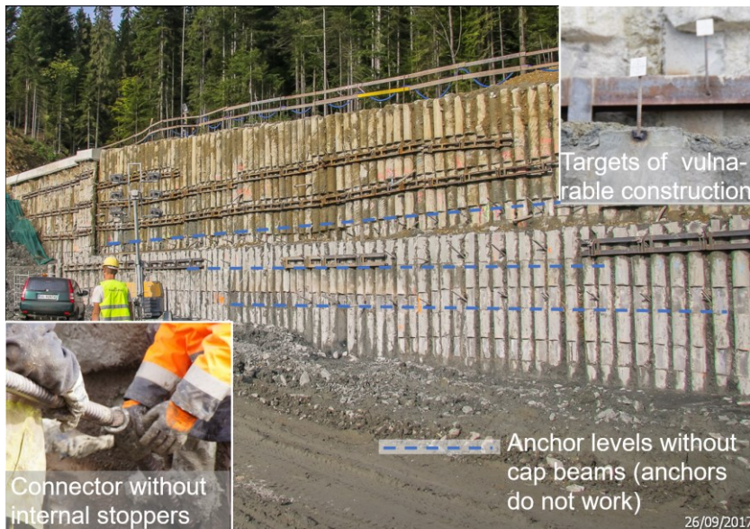
Fig. 3. View of the retaining wall with presentations of some of the execution errors.
